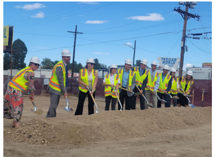
Fax Executive Director Monica Martinez lifts a shovel at the 7900 E. Colfax groundbreaking on October 6.
