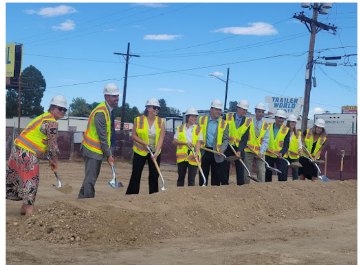
Fax Executive Director Monica Martinez lifts a shovel at the 7900 E. Colfax groundbreaking on October 6.
