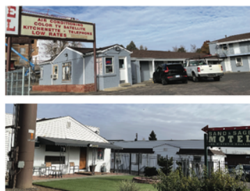
The Westerner and Sand & Sage motels were acquired by The Fax for temporary shelter space for families experiencing homelessness and affordable housing in the future.
